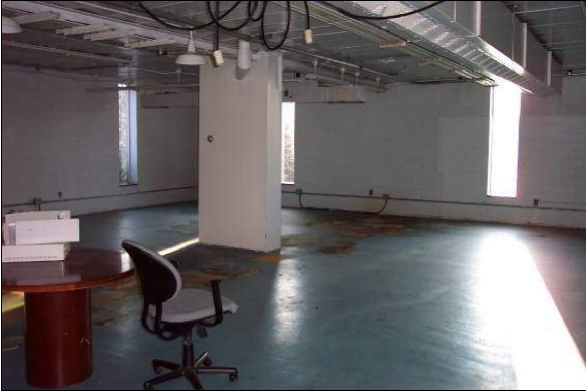
View of first floor of Building E
