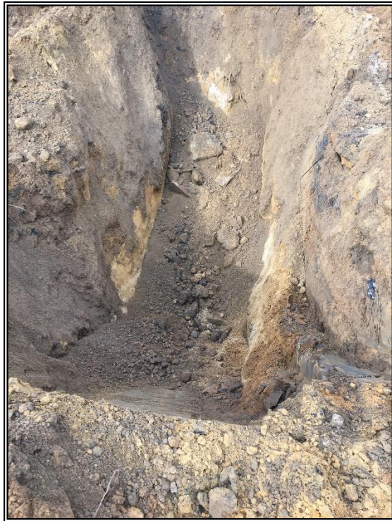
Photo 10: Anomaly Test Pit
